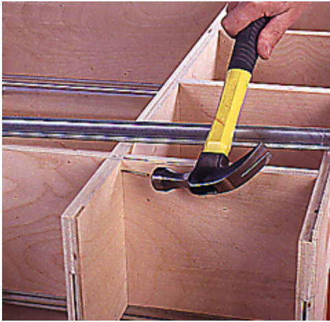
16--While holding the parts in position with clamps, drive a nail through the shelf and into the top of the inner side.
